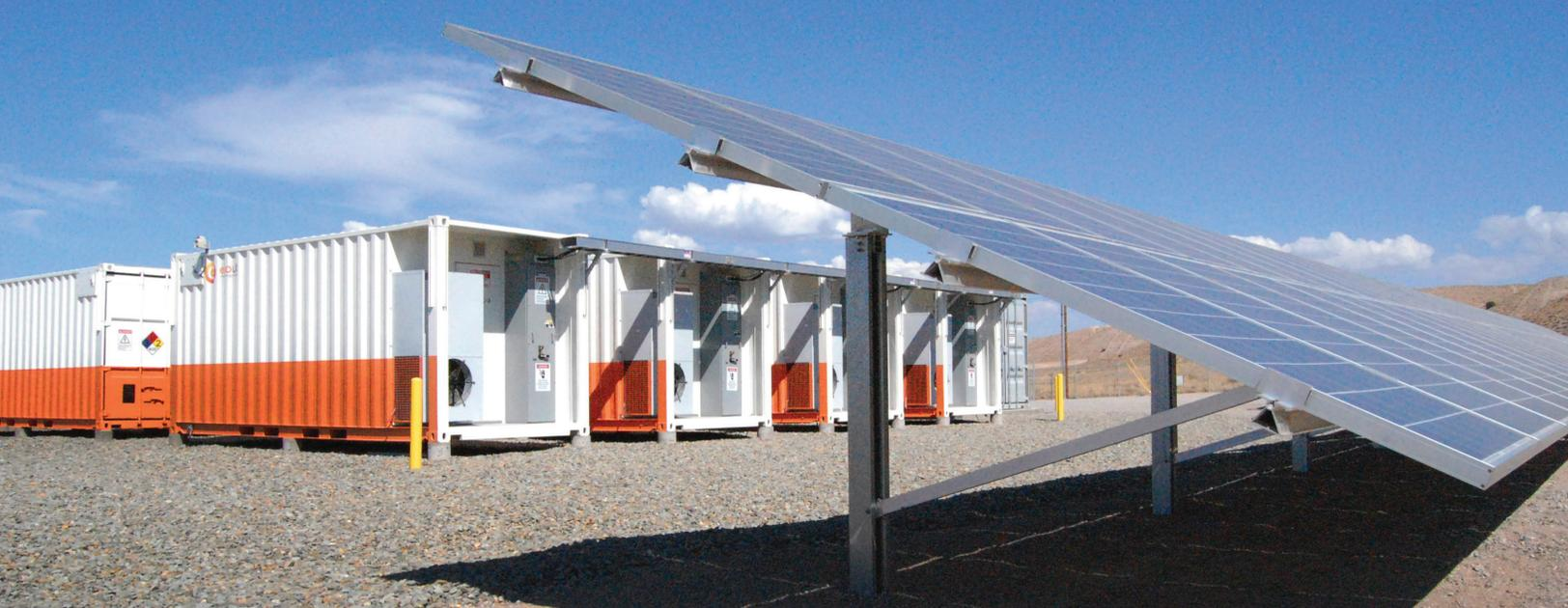
Public Service Company of New Mexico has a solar energy farm that uses lead batteries to effectively store solar input and regulate energy distribution.
