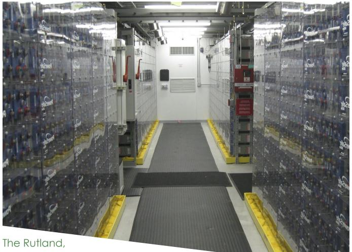
Vermont microgrid is comprised of solar panels, backed up by OptiGrid<sup>™</sup> Stored Energy Solutions by EnerSys<sup>®</sup>. It is the first solar microgrid funded by the U.S. Department of Energy (DOE) and the first system in the country that will be able to maintain mission critical power on renewables and storage alone for extended periods of time
